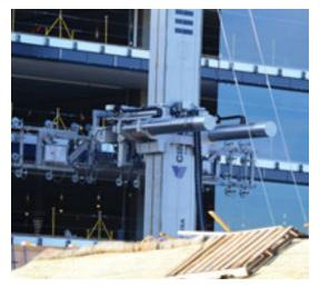
The huge walls of curved windows, claimed to be the largest pieces of arched glass ever made, are being installed with highly specialized machines like the one shown here.
